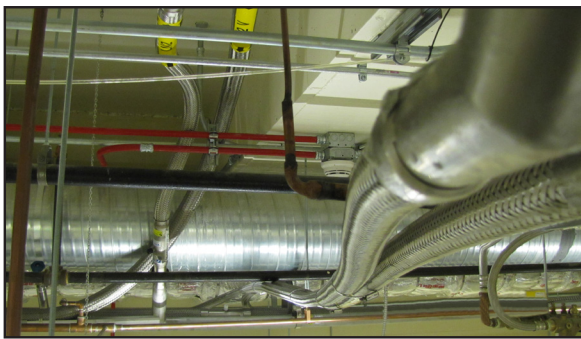
Engineer to Order Flex Pipe Installation
